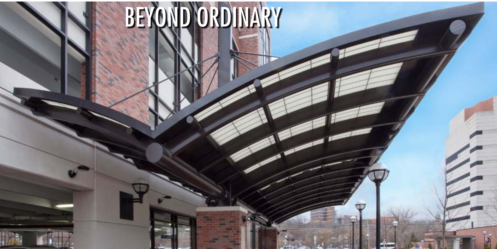
Parking Garage Canopy, Ann Arbor, MI, Walker Parking Consulting
