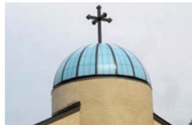
St. Mina & St. Abanoub Church, Miamisburg, OH, Bruns General Contracting
