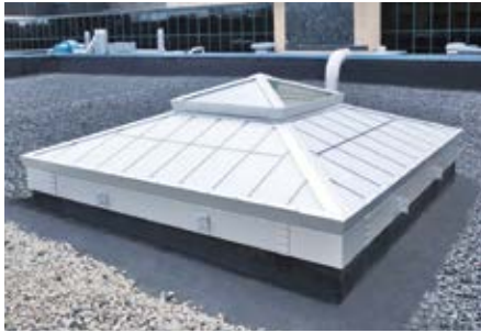
Above: Medical Center - Removable Skylight Over MRI Machine
